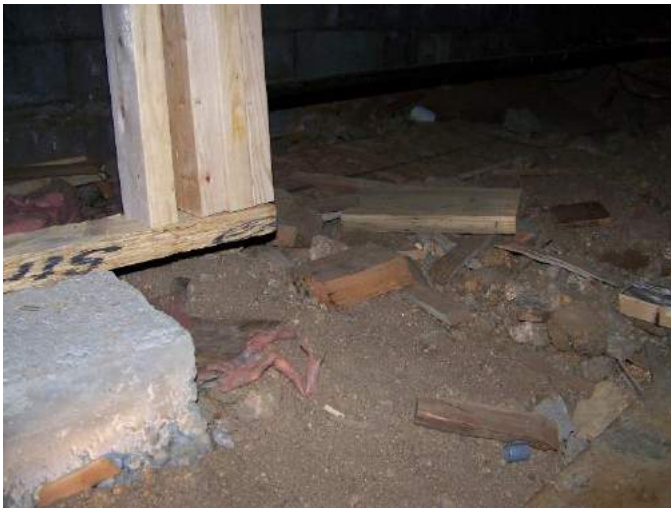
Missing point loads in the crawl space
