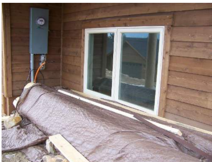
A blocked bedroom egress window. (2015 IRC sec. R310 Amend)
