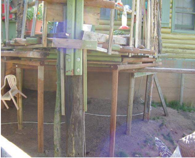
Unsafe deck beams, posts, footings, and rails.
