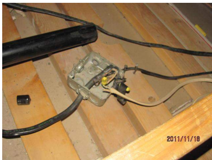
An accessible exposed electrical box.
