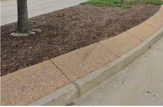
Sloped splash block design: existing Standard Arterial Streetscape corridors throughout the city include extensive segments with existing sloped concrete splash blocks, per a former standard.
