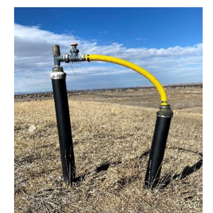
Landfill gas wellhead.
