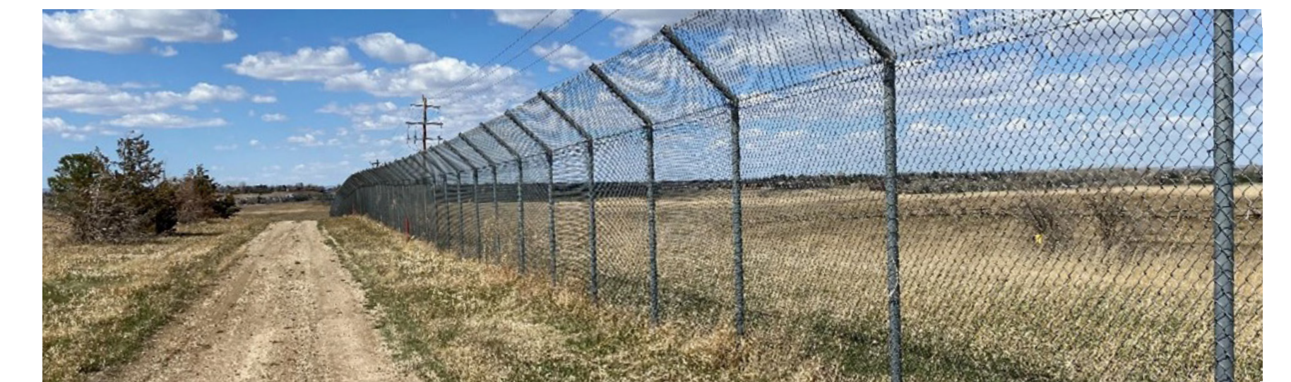
Site Perimeter Fencing.
