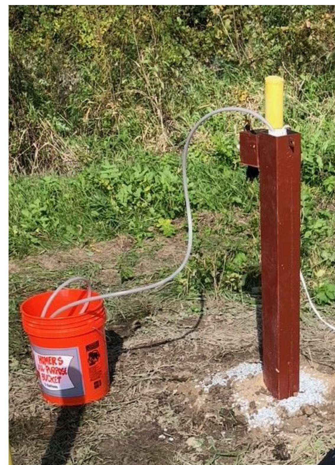
Groundwater monitoring well.
