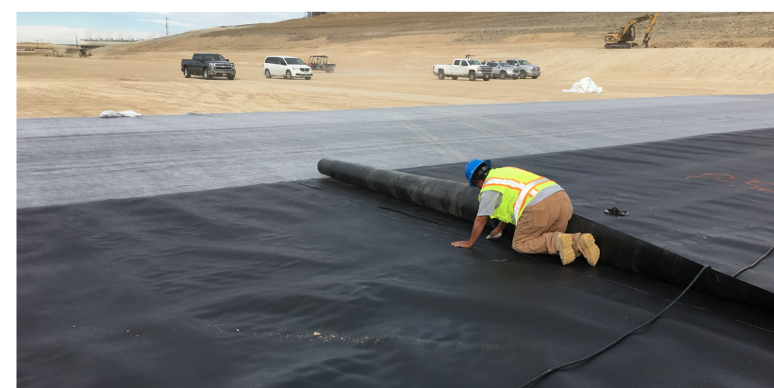
Installation of 60 mil HDPE Geomembrane Liner on geosynthetic clay liner and the prepared subgrade.
