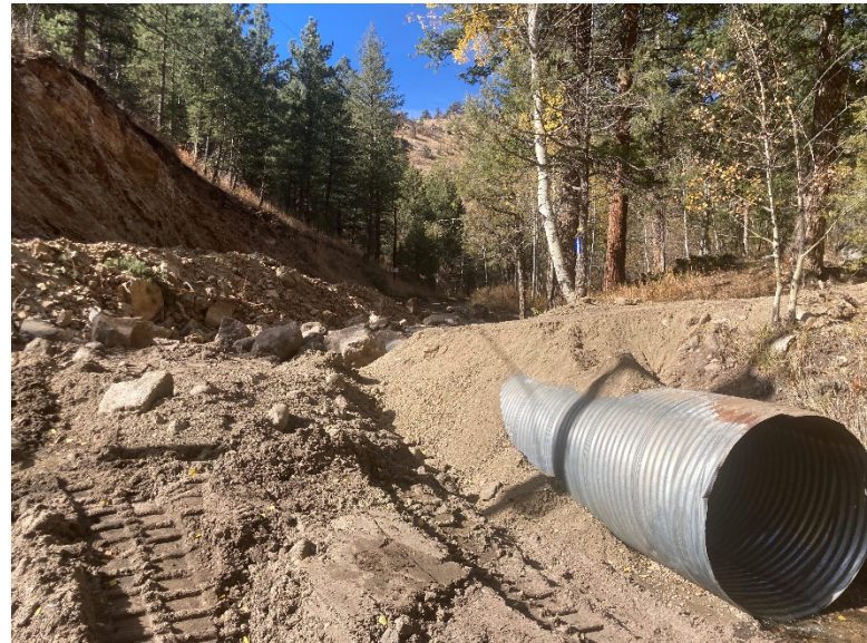
Figure 1- 48" Culvert at 436 Black Creek Dr
