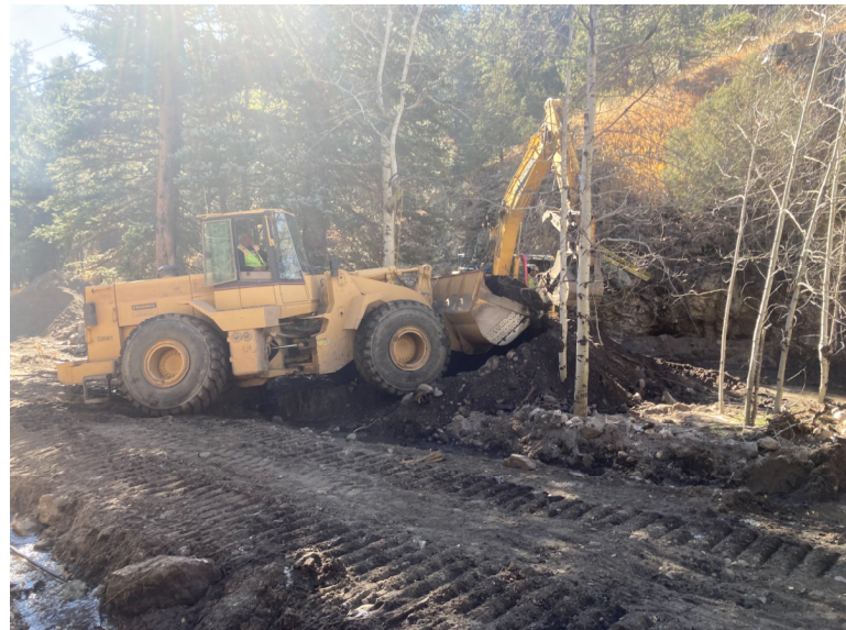
Figure 2- Removing deposited material from stream channel
