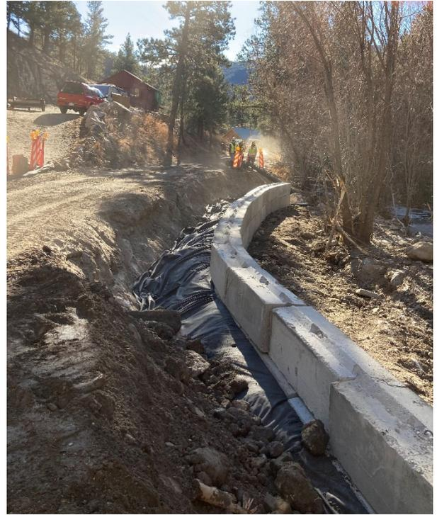
Photo 1- Revetment concrete block wall
