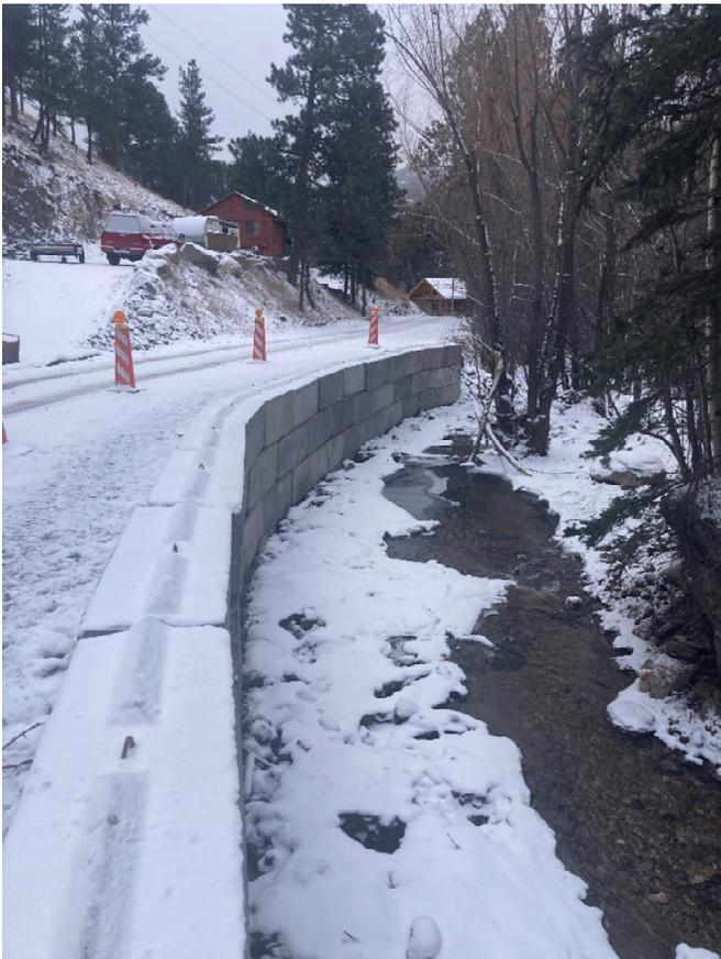
*Photo 4- Completed concrete block wall*
