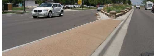
Tan exposed-aggregate concrete median paving.
