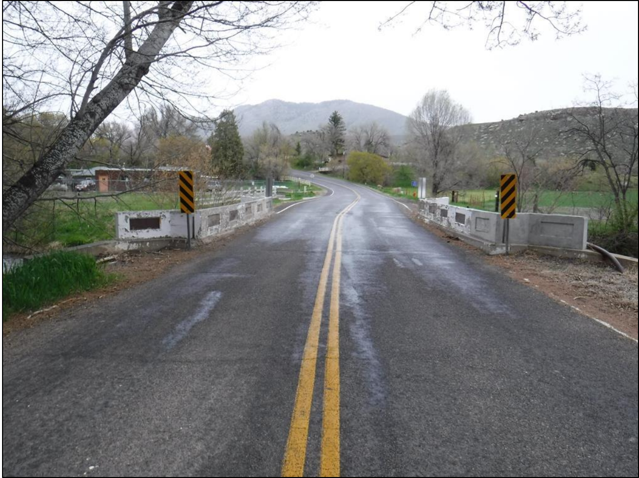
LR27-0.1-32C (Masonville Bridge) over the Buckhorn Creek Looking East
