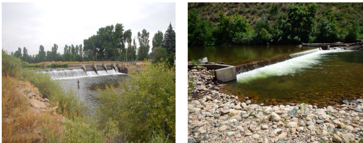
Figure 3.12: There are nineteen major structures or dams on the study area. Some pose major barriers for fish (left), while others are much lower and may be passable at some times of the year (right).
