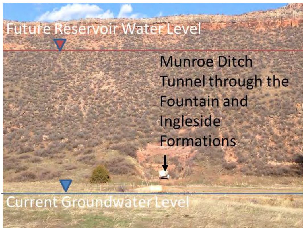
Figure 6 -Reservoir submergence of the Munroe Ditch tunnels leading to collapse
