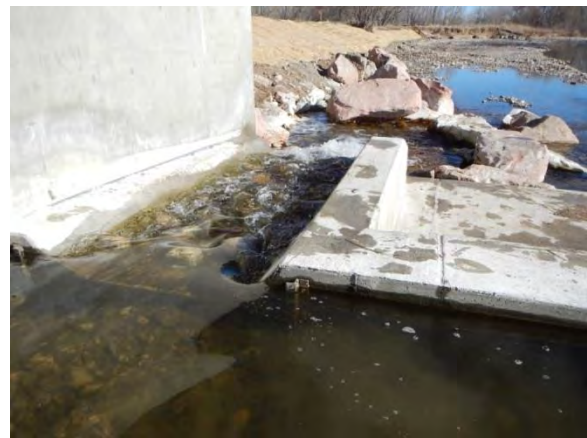
Figure 5.12: Recently installed fish passageway at the Fossil Creek Inlet Ditch just downstream of Prospect Avenue.
