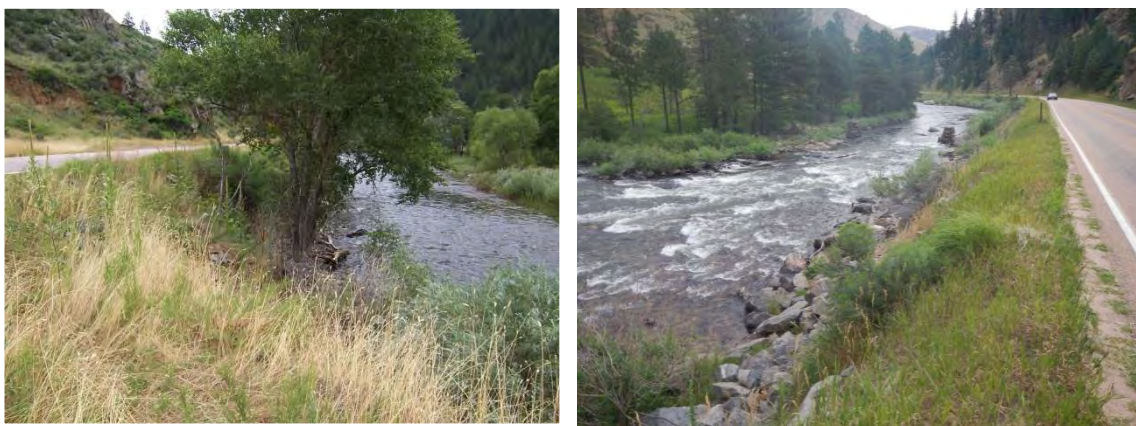
Figure 3.8: Highway 14 road fill encroachment in the riparian floodplain is common in the Canyon zone.
