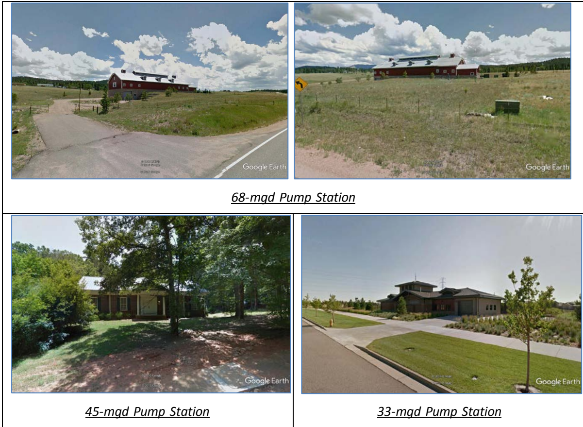
FIGURE 2.a-4 Example Pump Stations
