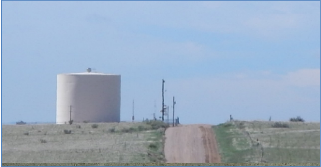
FIGURE 2.a-2 Example Appurtenance: Water Tank
