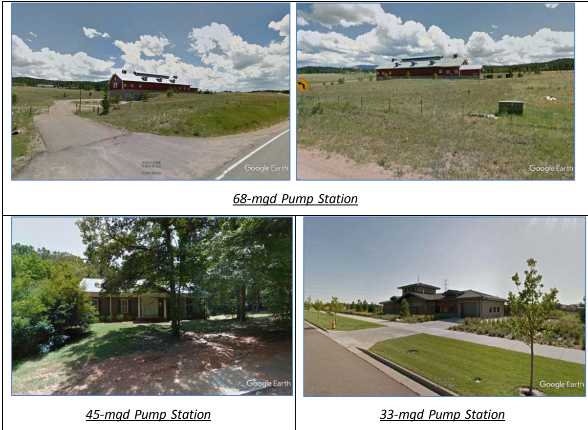
FIGURE 2.a-4 Example Pump Stations
