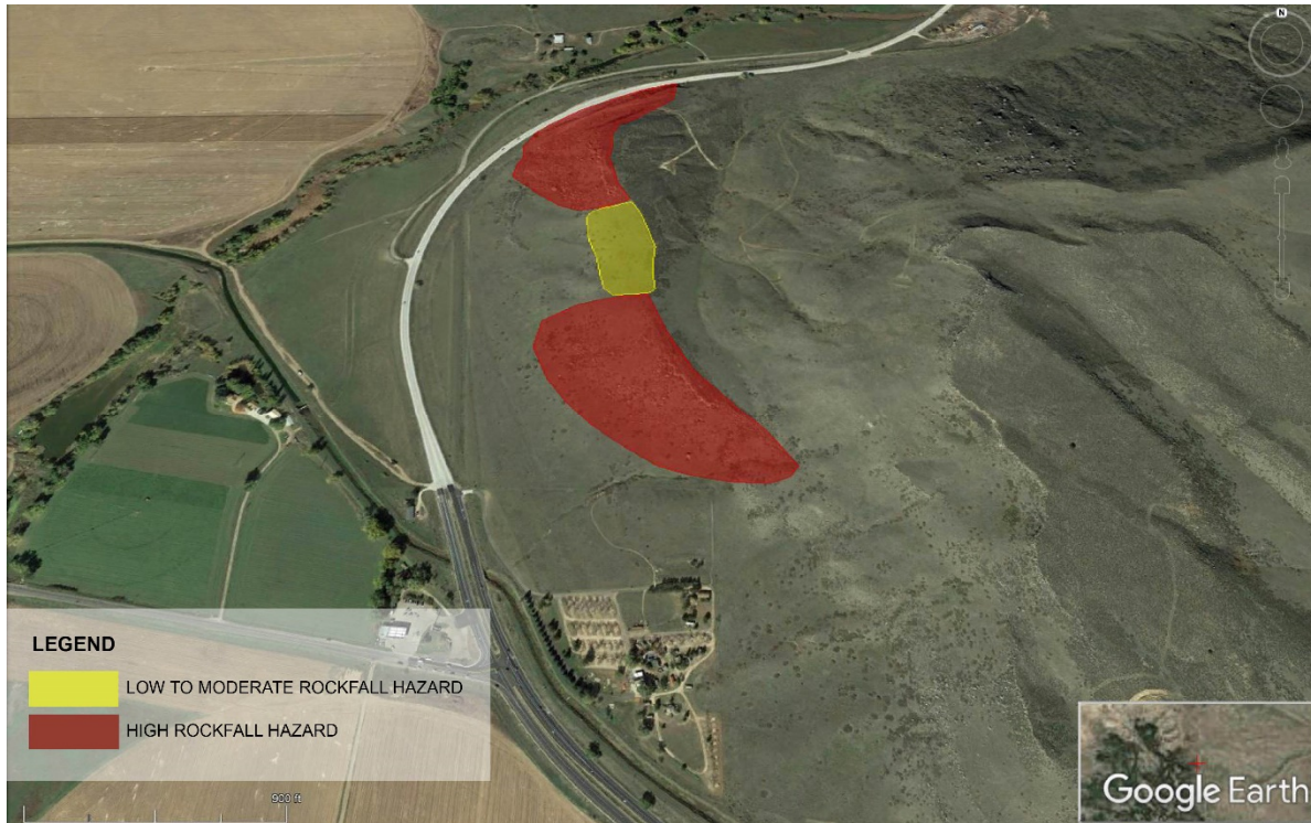
Figure 4 - Rockfall Hazard Zones
