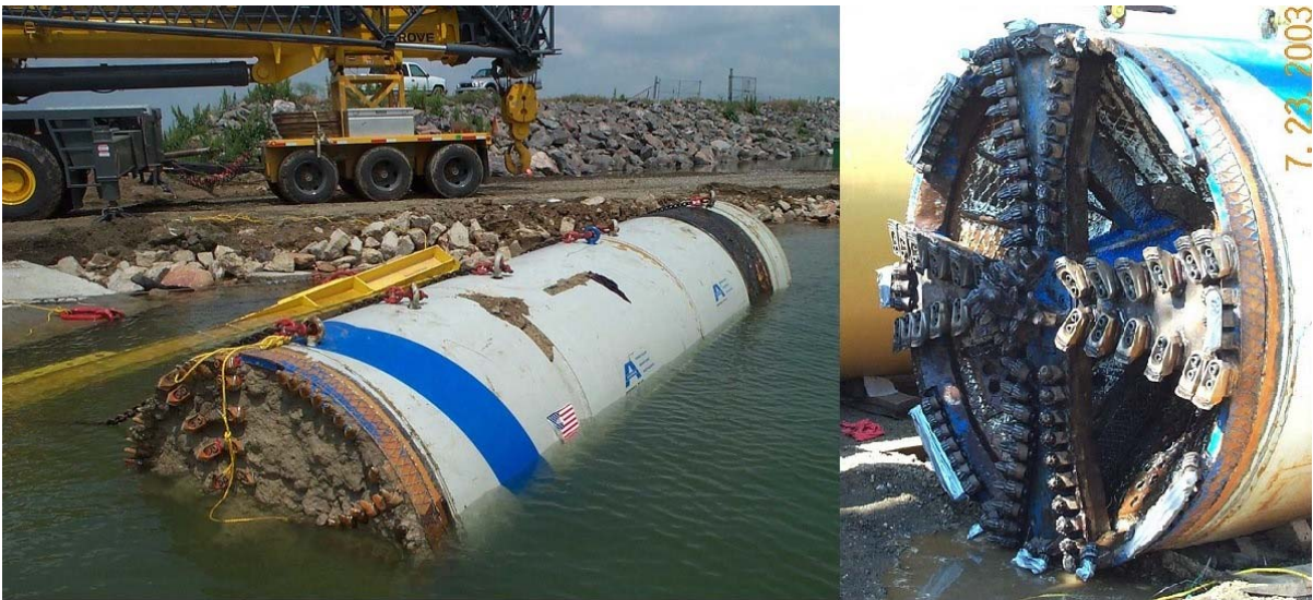
FIGURE 8 75-inch diameter Akkerman SL74 MTBM at Standley Lake Intake (Deere et.al 2005, Goss 2006, Jacobs files)
