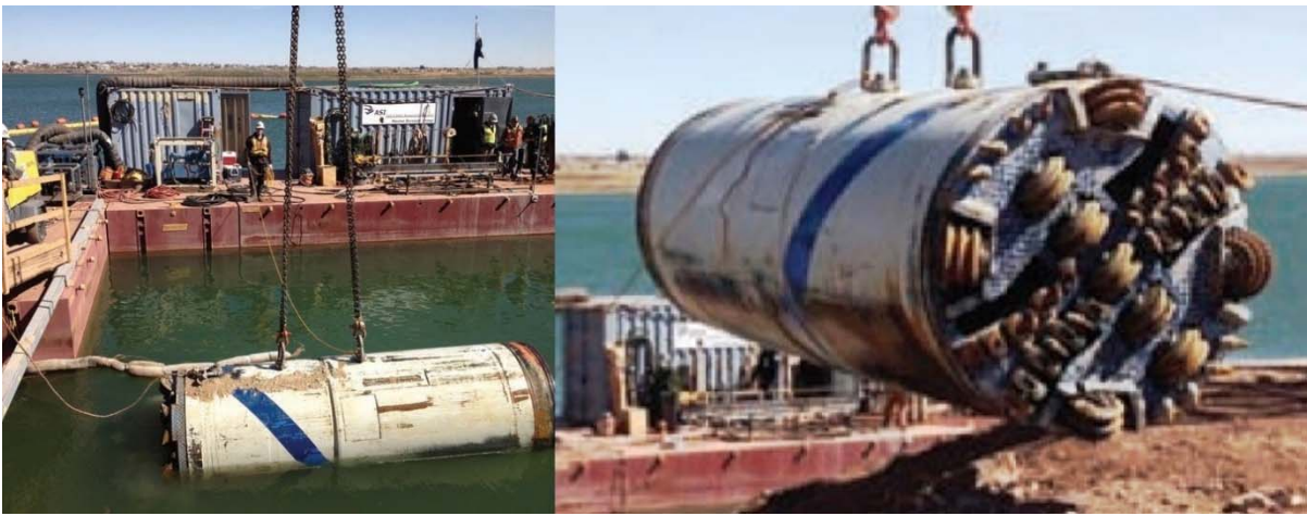
FIGURE 7 62.5-inch diameter Akkerman SL60 MTBM at Ute Reservoir Intake (Anderson 2014, Worthen et.al 2015)
