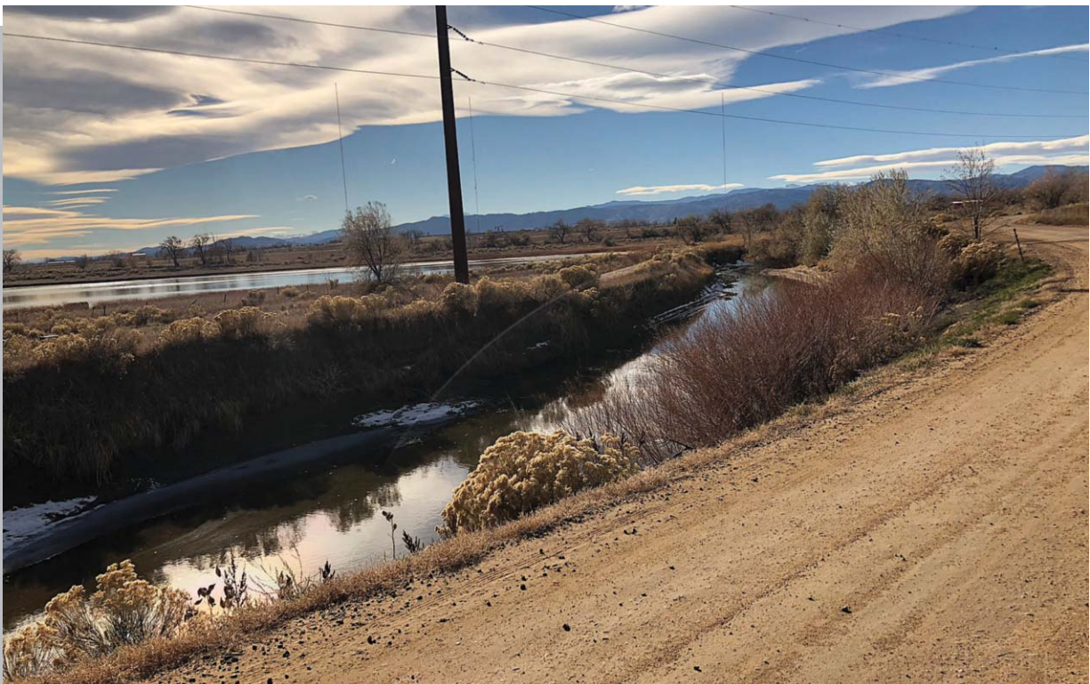
Photo 2 - Larimer County Canal running through the southern portion of the TWP additional analysis area, along the southern edge of East County Road 56. View is to the southwest.
