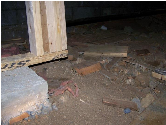
Missing point loads in the crawl space
