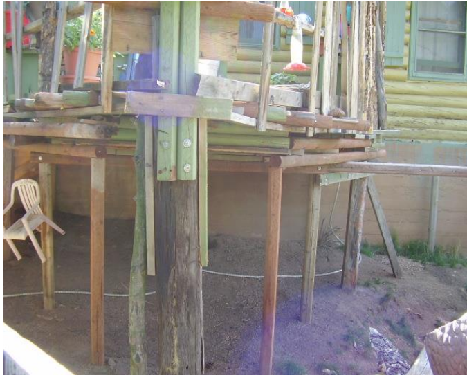
Unsafe deck beams, posts, footings, and rails.
