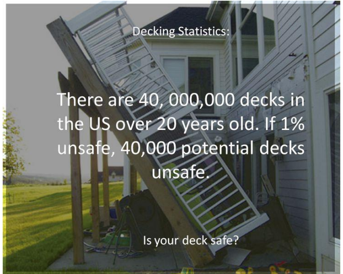
Unsafe connections to beam, ledger.
