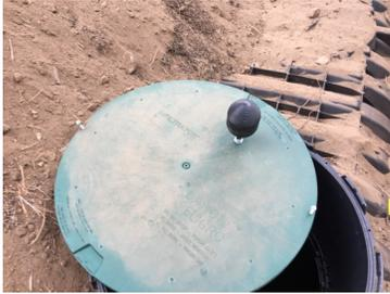
**Vault**-A minimum 1250 gallon watertight, sealed tank designed to store wastewater. Vaults must be equipped with a signaling device to indicate when they are reaching capacity and must be pumped when full.
