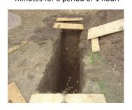
The site and soil evaluation is an important part of the permitting process for on-site wastewater treatment systems (OWTS). The site evaluation is used to determine if site and soil conditions are suitable for installation of an OWTS, the size of the soil treatment area, and if any physical features such as lakes, creeks, irrigation ditches, drainages, or wells may require setbacks to prevent possible contamination.
