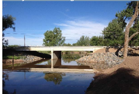
County Road 19 Bridge
