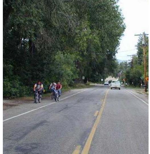
Narrow Shoulders for Bicycling
