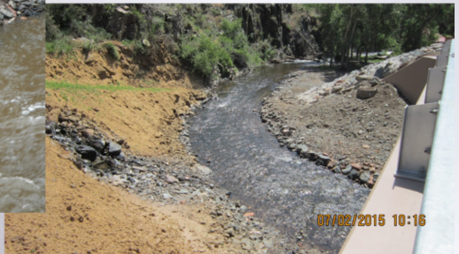
River restoration work on Buckhorn Road
