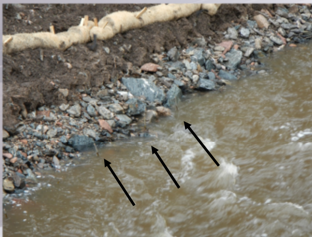
Willow poles planted along embankment
