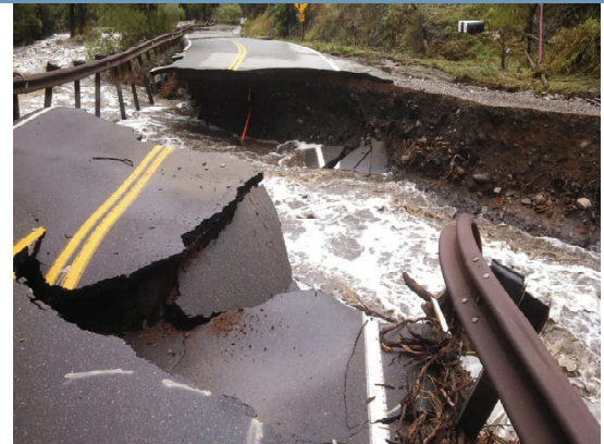
Flood Damage (CR 43 )
