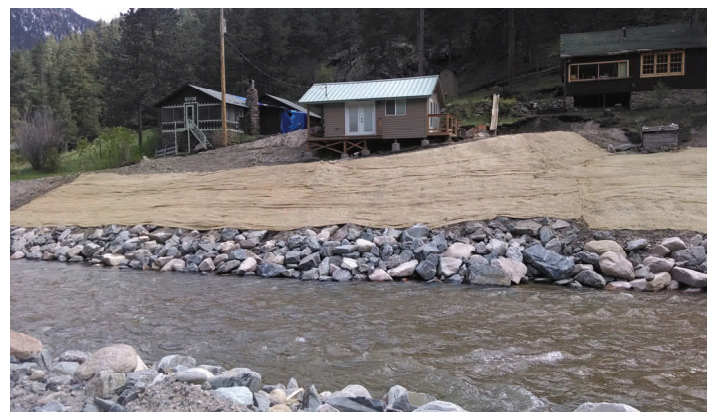
Final bank stabilization
