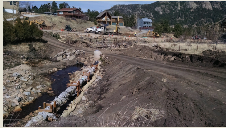
Fish Creek Utility Work
