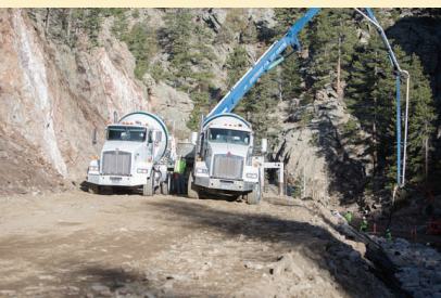
Grouting Riprap along the stream bed (CR 43)
