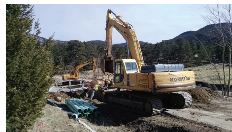
Utility work on Fish Creek
