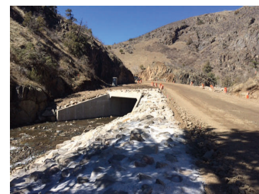
CR 27 bank stabilization
