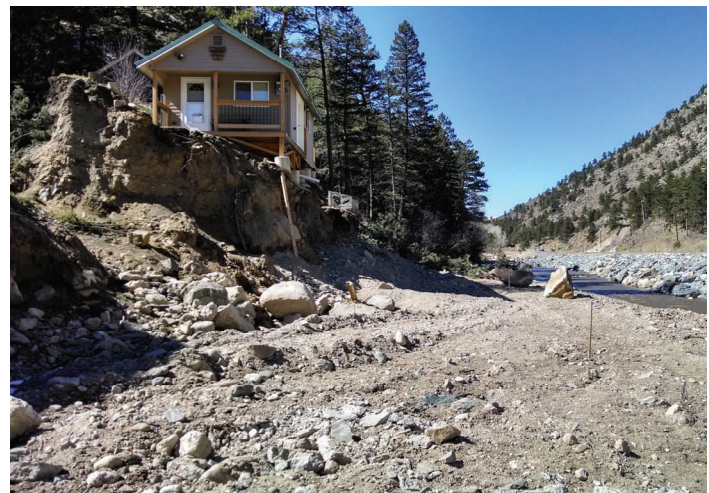
Flood damage in the Big Thompson Canyon
