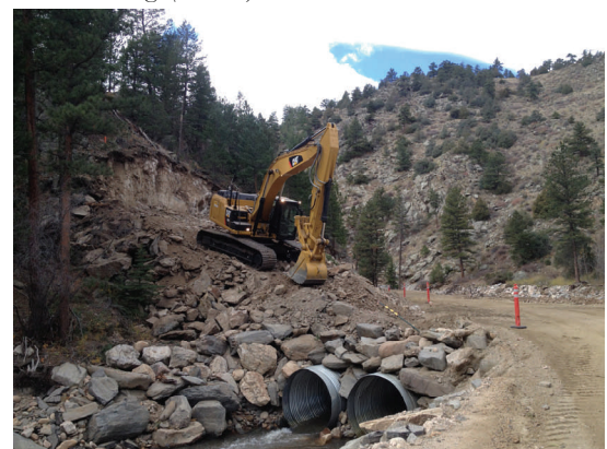
Temporary repairs (CR 43)
