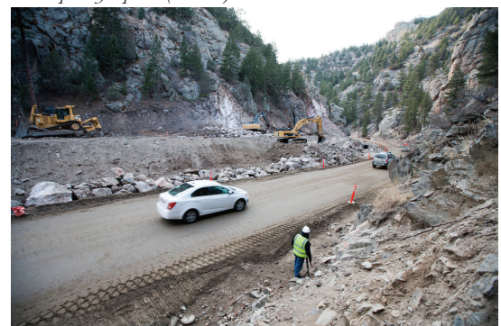
Permanent repairs into bedrock (CR 43)
