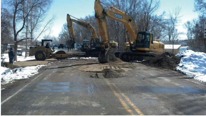
An old wooden bridge on County Road 54G over the Jackson Ditch was replaced. (Photo: Gabe Routzahn)
