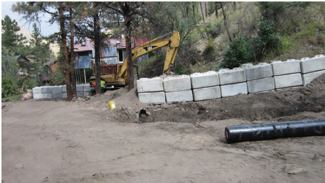
Large concrete blocks were installed in areas affected by the High Park fire to redirect debris and runoff flows and protect property.
