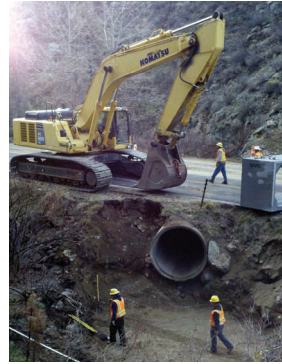
Installation of large box culverts was completed on Rist Canyon Road (CR 52E). (Photo: Gabe Routzahn)
