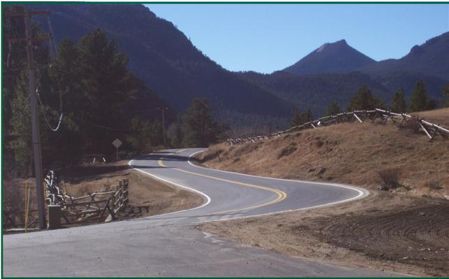
Two culverts were replaced on CR 43 and a minor realignment was completed. Photo: Frank Kurtyka
