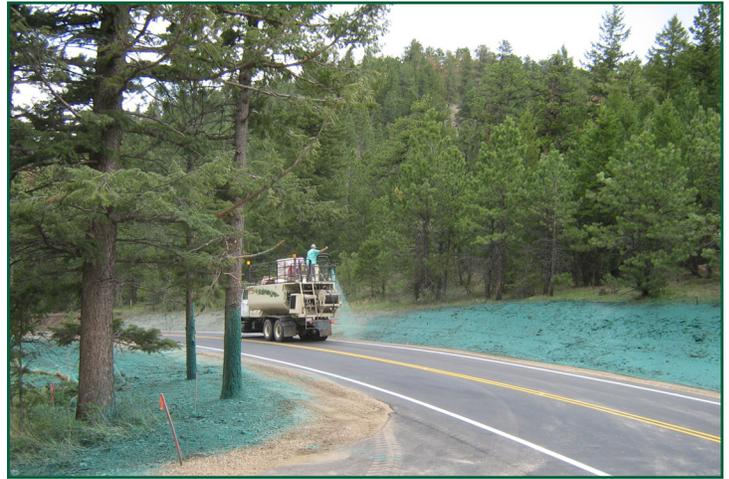
Hydromulching as final construction step on CR 27 as a safety project is completed. The application of seed, fertilizer and moisture retention encourages grass growth and reduces erosion. Photo: Preston Pierson
