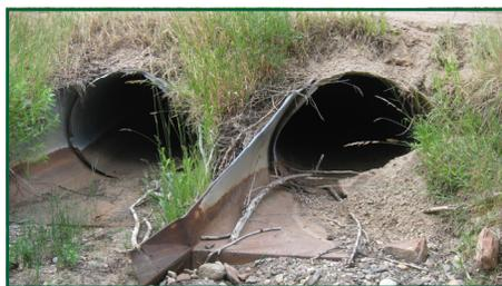
*A series of seven old and small sized culverts passing Rist Creek underneath CR 52E (Rist Canyon Road) are being replaced with large box culverts. The new culverts have more capacity, are less susceptible to clogging by debris, and are designed to protect the roadway from washing out as much as possible.*
