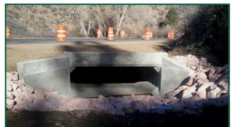
and the area around the culverts are armored to protect the road should overtopping occur.
