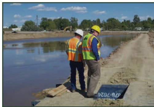
Sediment from the reservoir was pumped in pipes more than a half-mile to large ponds for dewatering. Photo: Mark Peterson
