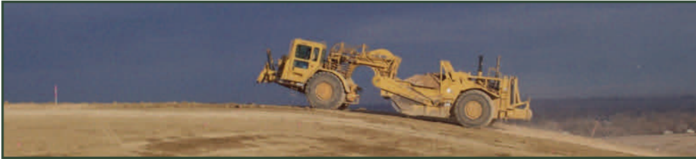
Engineering Department provided engineering design and construction management services to the Solid Waste Department for the closure of the most recent cell at the landfill. Photo: Frank Kurtyka
