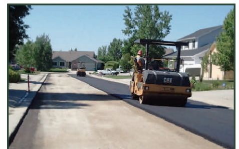
The Crown Point subdivision in North Loveland used funding in its Public Improvement District (PID) to complete road reconstruction for its neighborhood streets. Photo: Matt Johnson
