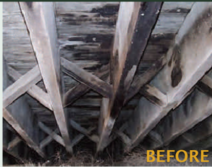
The CR 7 bridge over the North Poudre Inlet Canal was an old timber structure that had become structurally deficient. The new bridge is constructed out of concrete box girders. Photo: Ron Winne
