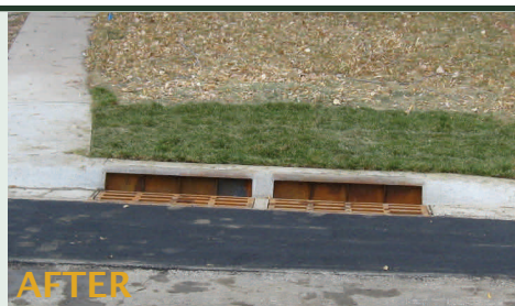
This is an example of a storm drain enhancement completed as a part of a subdivision road improvement project funded through a Public Improvement District. Photo: Matt Johnson
