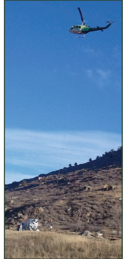
Helicopter placement of concrete for new transmission lines for the Platte River Power Authority included construction access permitting through the Engineering Department. Photo: Darrell Morrell
