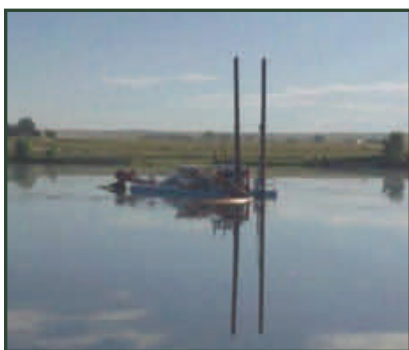
The dredge equipment to remove sediment from Clark Reservoir was trucked in from the east coast. Photo: Preston Pierson
