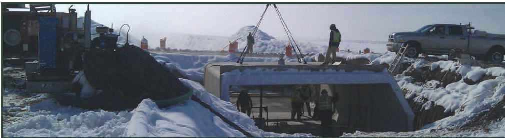
The placement of the new box culverts on CR 42E over two canals had to be completed during the off-season for irrigation. Photo: Preston Pierson
