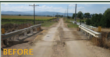
CR 42E crosses over a pair of irrigation ditches just east of CR 5. The old crossings were badly deteriorating wooden structures with rotting wooden piles. The new structures are concrete box culverts. Photo: Preston Pierson
