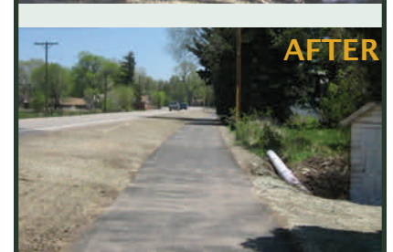
County Road 54G through the town of LaPorte had a very poor pedestrian trail with grated crossing over a canal. Through a partnership with the Department of Natural Resources and with support from Poudre School District, the Engineering Department was successful in getting federal transportation enhancement funds to replace the structure and complete the trail, which will also serve as a part of the Poudre River Trail system. Photo: Kyle Arend
