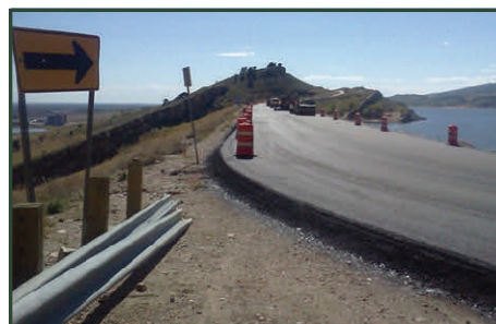
CR 23 along the east side of Horsetooth Reservoir was overlaid to address road maintenance issues. The Bureau of Reclamation provided funding for additional asphalt over the dams to even out dam height elevations. Photo: Marc Lyons
