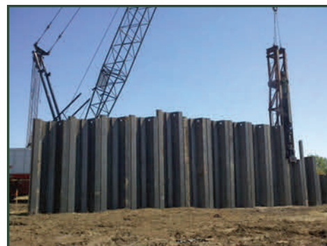
A sheet pile retaining wall was pounded into the ground to channelize the inlet canal. Photo: Preston Pierson
