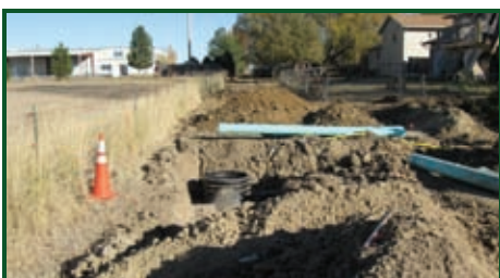
Drainage work in an Improvement District was funded by local residents. Photo: Matt Johnson
