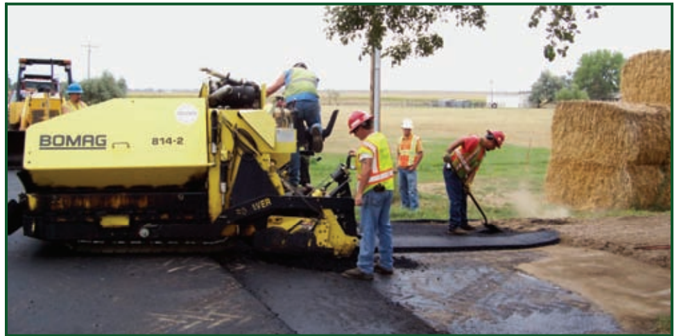
Asphalt paving often includes paving driveway approaches to private properties. Photo: Marc Lyons
