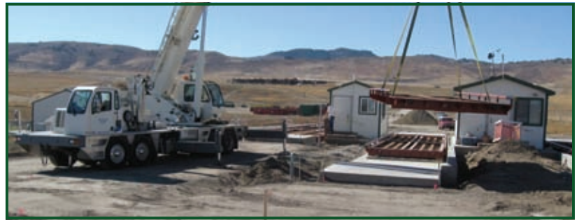
To meet new EPA mandates, the Larimer County Landfill was required to install scales to monitor the weight of materials brought to the site. The Engineering Department assisted the Solid Waste Department with the scale design, traffic circulation and construction management. Photo: Matt Johnson
