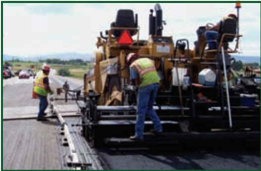
The approach to a railroad crossing on CR 30 is reconstructed to provide for a smooth traveling surface. Photo: Marc Lyons
