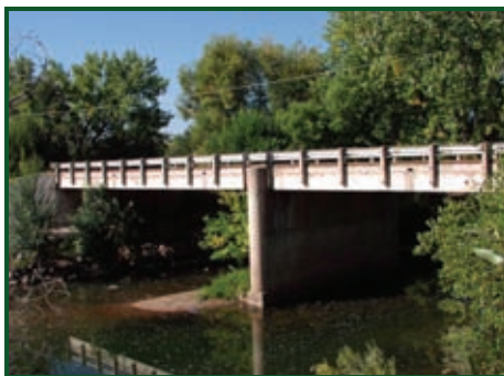
The CR 17 (Shields Street in north Fort Collins) bridge over the Poudre River will be replaced using a federal bridge grant. Photo: Ron Winne
