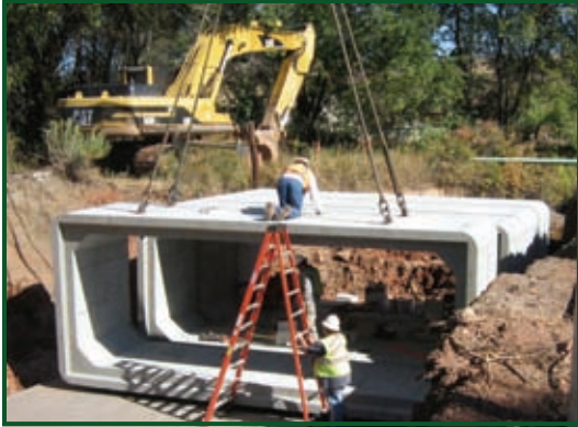
A large concrete box culvert was placed under CR 19 in order to maintain historic water flow paths under the road. Photo: Marc Lyons
