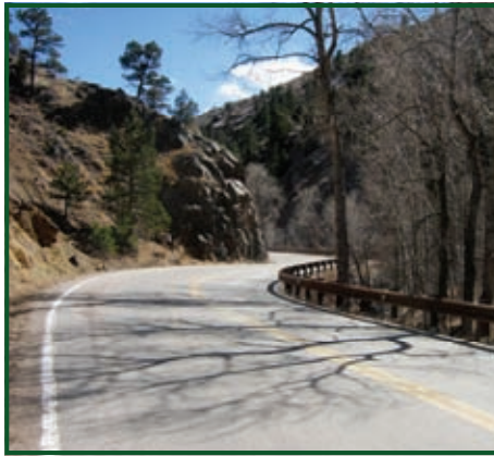
The installation of guardrail along a section of CR 27 with higher than typical accidents was funded by a federal Hazard Elimination and Safety grant. Photo: Preston Pierson
