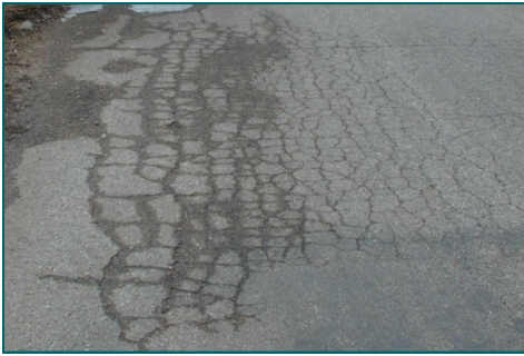
It is much less expensive to maintain pavement than rehabilitate it once it has failed. Photo: Engineering Staff
