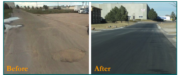
During 2008, the Centro Business Park completed more than $ 1/2 million dollars of badly needed maintenance and road reconstruction through their newly created Public Improvement District. The work significantly improved the safety, mobility and accessibility in this commercial and industrial area. Photo: Matt Johnson
