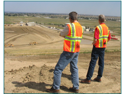
Overseeing construction work on the completion and closure of a section of the Larimer County Landfill. Photo: Rusty McDaniel
