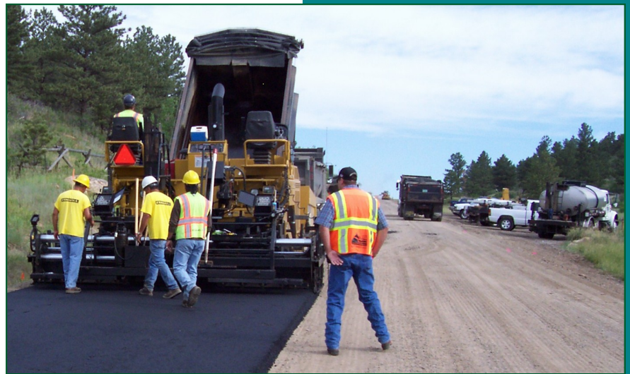
Overseeing asphalt work on CR 23 (Centennial Drive) near Horsetooth Reservoir. Photo: Marc Lyons
