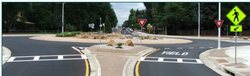
Larimer County's first modern roundabout at the intersection of Taft Hill Road and Vine Drive. The long backups of years past are gone, the number and severity of accidents at the intersection are dramatically reduced, and 85% of survey respondents now support the roundabout. Photo: Kyle Arend
