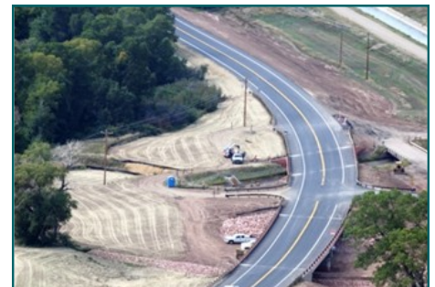
New bridges on CR 38E in the Masonville area addressed structural, stormwater and safety concerns. Photo: Charlie Johnson
