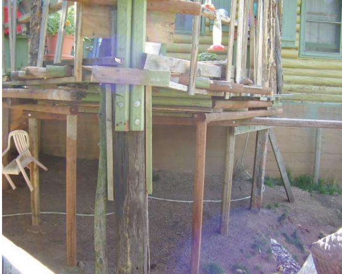
Unsafe deck beams, posts, footings, and rails.
