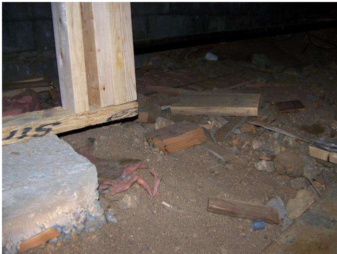
Missing point loads in the crawl space
