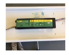
2. Cut wires leading from ballast on both sides.
